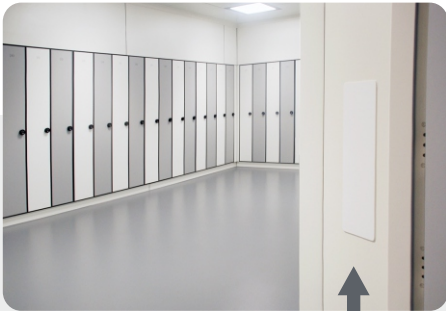
Antennas in the primary changing rooms detect unauthorised return of persons wearing cleanroom clothing.
