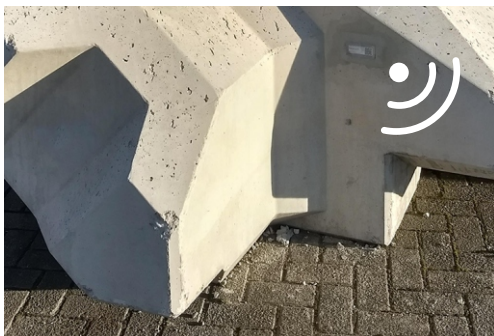
Level-bloc with embedded RFID tag containing the product information.
