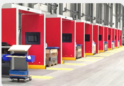
12 RFID portals detect incoming and outgoing pieces of furniture
